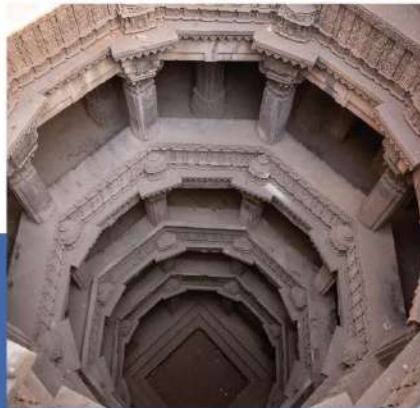
Fig. 1. The octagonal structure of Bal Hari ni Vav, a stepwell commissioned in 1485 by the homonymous woman, Ahmedabad, Gujarat. © Somya Parkh, 2019 - Living Waters Museum.
