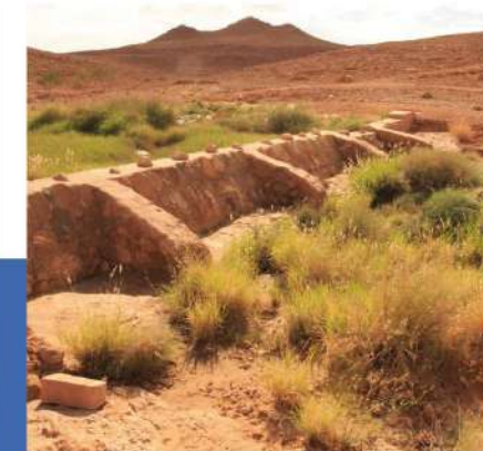
Fig. 4. Re-adaptation of dykes in the new agricultural lands aims at recharging groundwater and recovering sediments as organic fertilizer. (photo by Farah Hamamouche).
