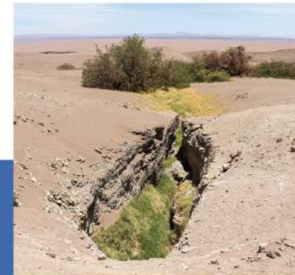
Fig. 4. Exit point of Santa Rosita. Despite being abandoned, sometimes water continues to flow out of the socavones and feeds vegetation in the desert. © Fundación Carpe Science.
