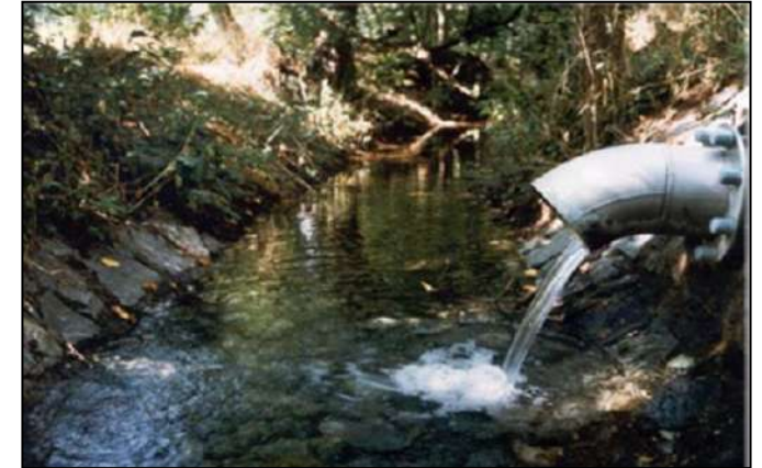
Former drainage trenches, now used for infiltration
