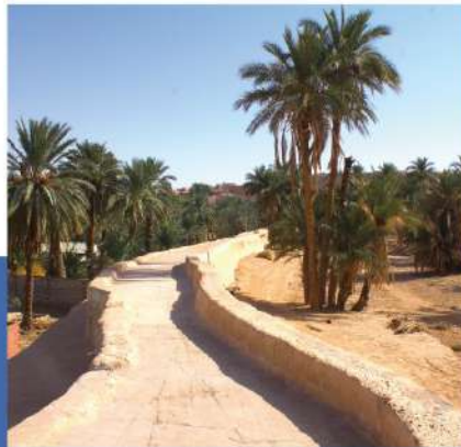
Fig. 1. The ancestral dyke built downstream of the Ben Isguen palm grove is functional to stop flood waters and recharge the aquifer. (photo by Farah Hamamouche).
