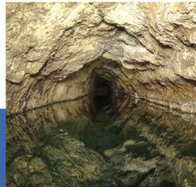
Fig. 3. The narrow gallery of San Isidro still with flowing water. However, due to the lowering of the aquifer level, today water does not reach the land surface. © Fundación Carpe Science.
