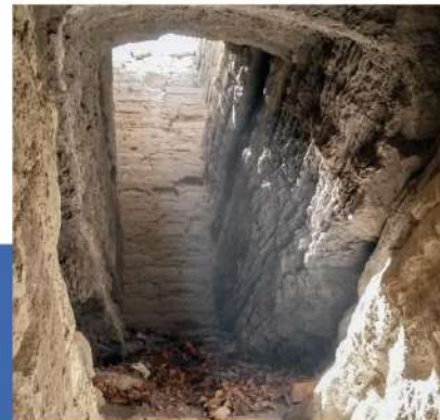
Fig. 2. Ventilation well ( lumbreira ). In Pica-Matilla, the lumbreiras are not vertically aligned with the main gallery. © Fundación Carpe Science.
