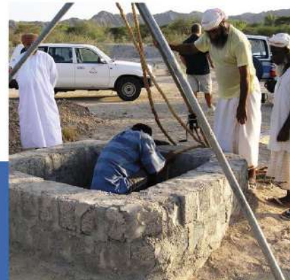
Fig. 3. Maintenance of the mother-well of the Daris falaj in Nizwa (World Heritage list of UNESCO). © University of Nizwa.
