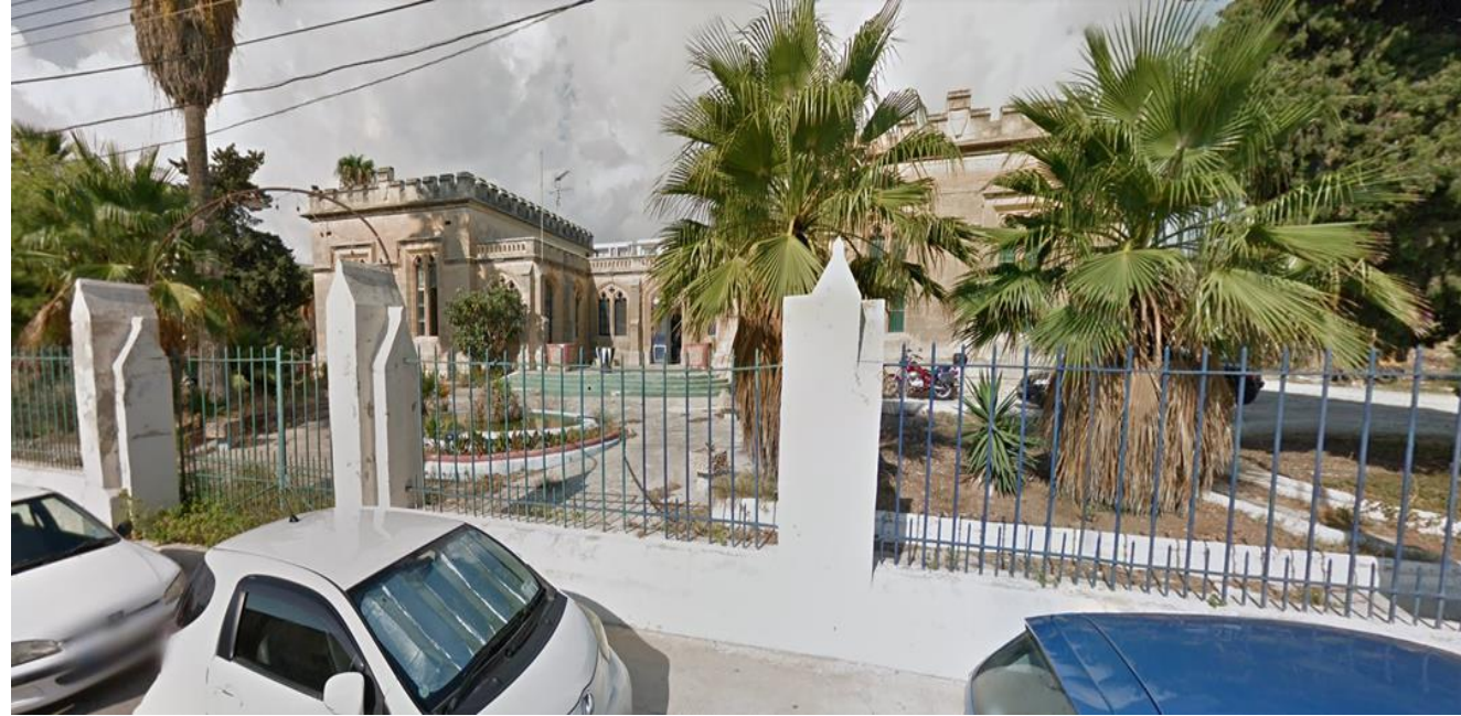
Wastewater Pumping Station
