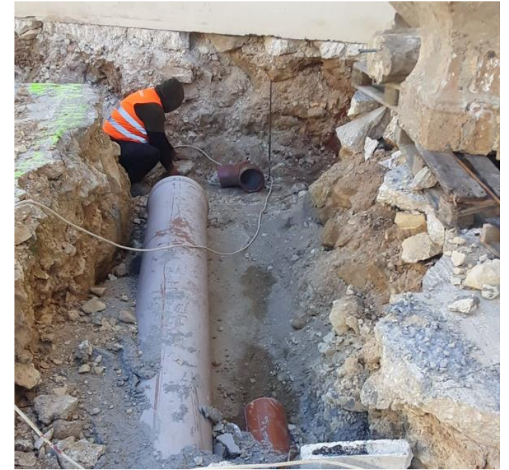
Storm Water installed next to Sewage Network {Dual Network}
