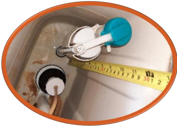
Setting the flushing cistern water level
