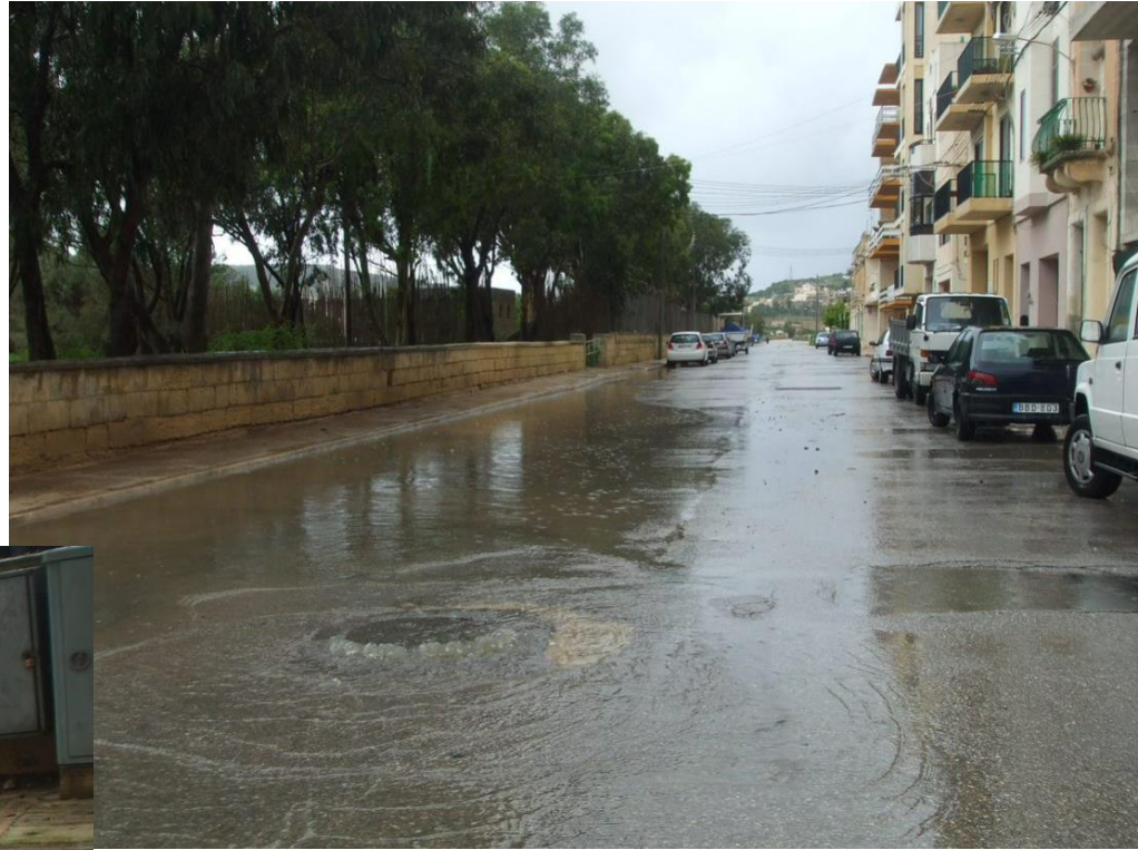
Overflowing sewage & rain water in street & ending up into 3 rd party property
