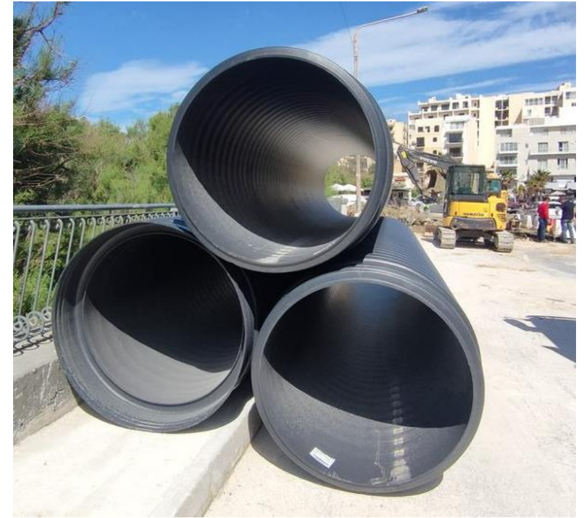
1.2m Storm Water Pipe being installed
